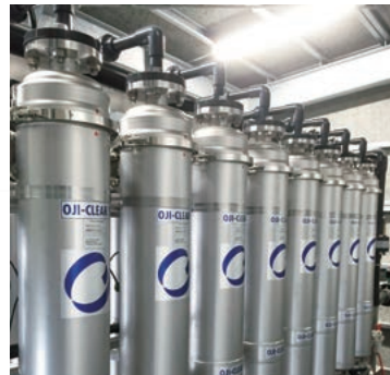
Water treatment system
