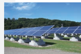
Oji Green Energy Shiranuka (Solar power)
