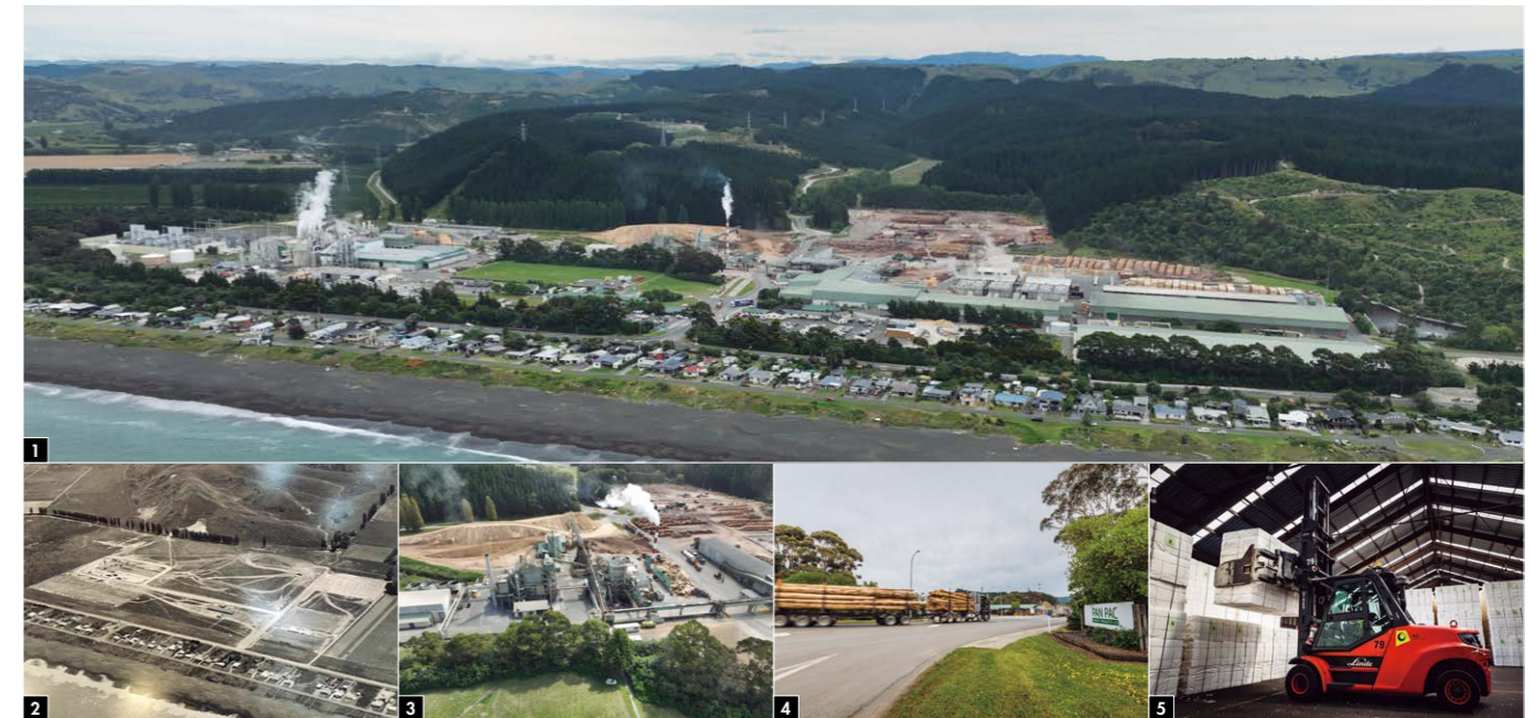
1 Current Pan Pac. Pulp mill (on the left), lumber mill (on the right), and Pan Pac's own forest (in the back). 2 Pan Pac in 1971. Aerial view of the mill when it was first built. 3 Biomass boilers. Steam is generated from wood chips and other materials produced in the lumber production process and used in the drying process of lumber and for in-house power generation. 4 Logs being delivered by log truck. 5 Warehouse at the port of Napier, a shipping port. Pulp is loaded onto the ship by a clamp lift.
