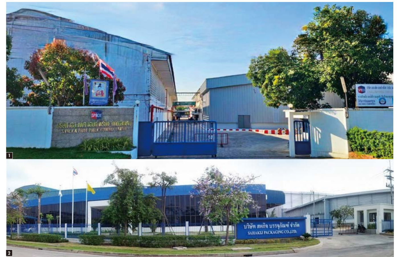
1 Front of S.PACK Mill 2 Front of Sahakij Mill
