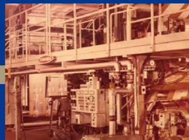
Installation of flexo rotary press
