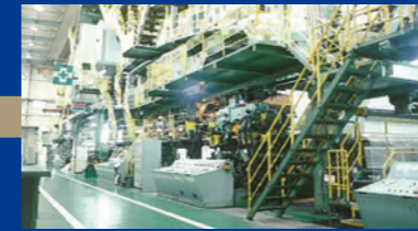
Kanzaki Paper started operation of No. 4 KS coater
