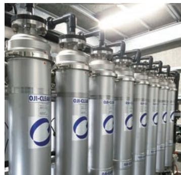
Water treatment system
