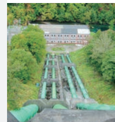
Oji Paper Tomakomai Mill Chitose No. 1 Hydroelectric Power Plant
