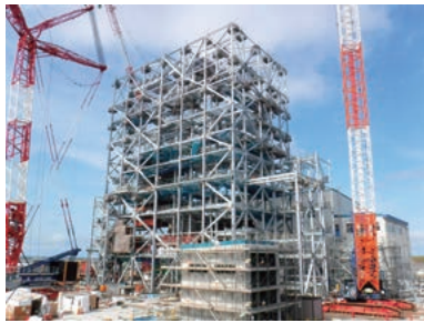
Biomass power plant under construction MPM Oji Eco-Energy (Hachinohe City, Aomori Prefecture)
