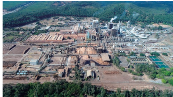
Overall view of the CENIBRA Mill (Belo Oriente, Minas Gerais, Brazil)
