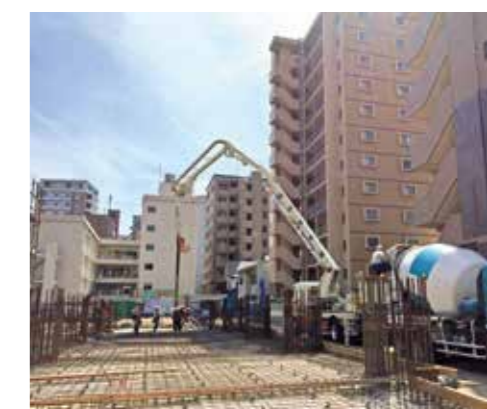
A concrete pump truck pumping concrete
