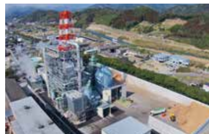
Biomass power plant (Oji Green Energy Nichinan/Nichinan City, Miyazaki Prefecture)
