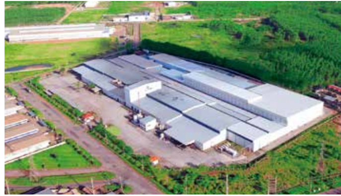
Overall view of the Oji Paper (Thailand) and Oji Label (Thailand) Plant
