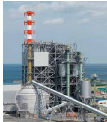
MPM Oji Eco-Energy's biomass electric power generation facility
