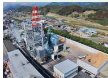
Biomass power generation
