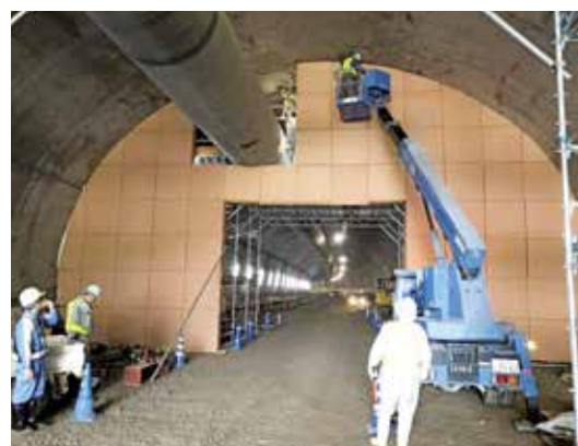
New construction method using HiPLE-ACE
