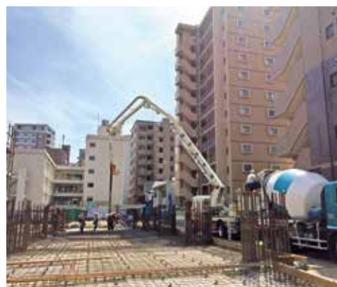
A concrete pump truck pumping concrete
