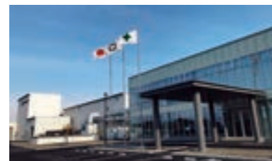
The new corrugated container plant in Funabashi City, Chiba Prefecture
