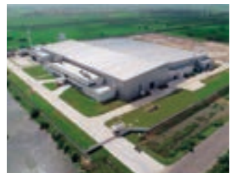
New corrugated container plant in Ahmedabad, Gujarat, India
