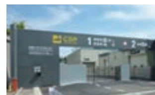
Confidential document processing facility (Oji Materia Edogawa Mill)
