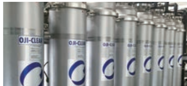
Waste water treatment system
