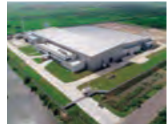
New corrugated container plant in Ahmedabad, Gujarat, India
