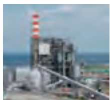
MPM Oji Eco-Energy's biomass electric power generation facility
