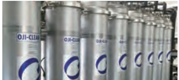
Waste water treatment system
