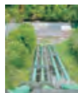
Oji Paper Tomakomai Mill Chitose No. 1 Hydroelectric Power Plant
