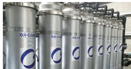
Water treatment system
