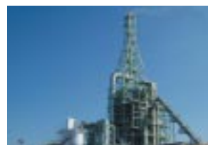
Oita Mill's RPF boiler
