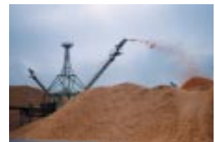
Tomakomai Mill's chip yard
