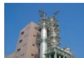
Kasugai Mill's continuous digester
