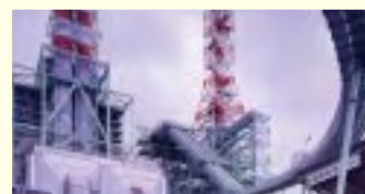
Yonago Mill's new-energy boiler
