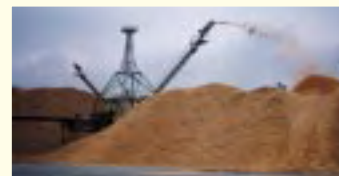
Tomakomai Mill's chip yard
