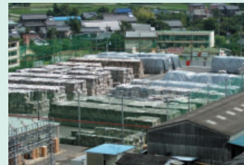
Recovered paper collection and stockpiling yard at the Sobue Mill
