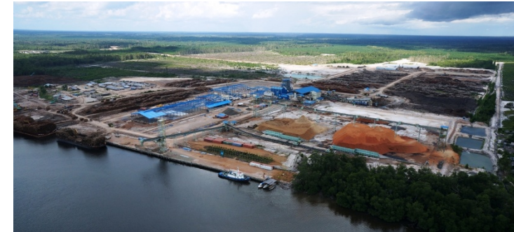
KTH mills in Natai region (chip mill, lumber mill, pellet mill, in-house power generation boiler, etc.)
