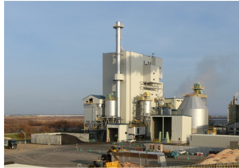
Oji Green Energy Ebetsu (biomass boiler under trial operation)
