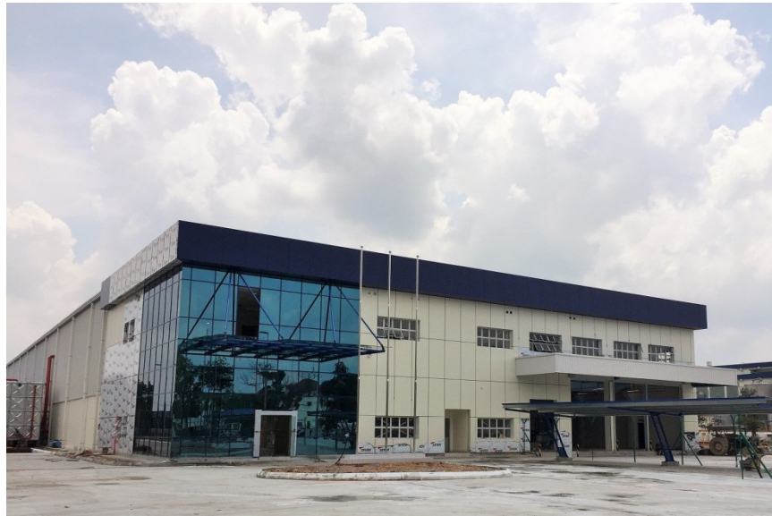
New disposable diaper factory being constructed in Malaysia
