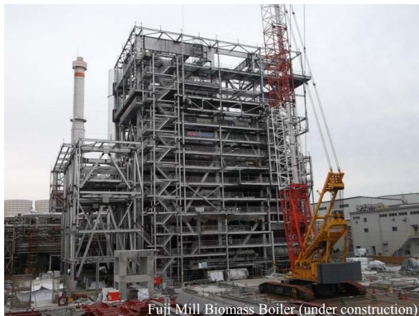
Fuji Mill Biomass Boiler (under construction)
