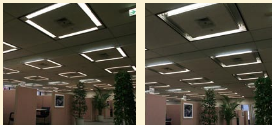
Before (left) and after (right) taking energy conservation measures with lighting. Covers were removed to maintain the needed illumination after the number of fluorescent bulbs was reduced (implemented in offices in the main building).
