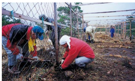
Building a drainage ditch on the restoration experiment site
