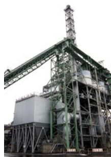
Photo 1 The new energy boiler put into operation in 2006 at the Nichinan Mill
