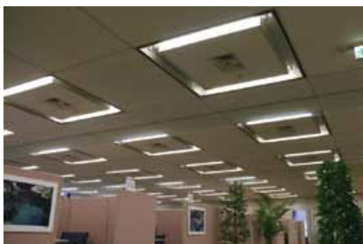
Partial removal of fluorescent lights
