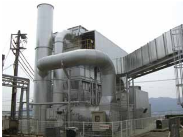
Deodorizing equipment (New Tac Kasei Co., Ltd. Toyonaka Mill)
