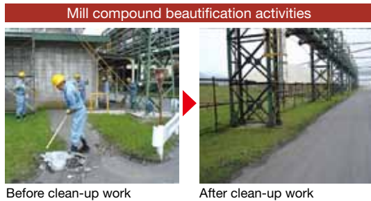
Before clean-up work
