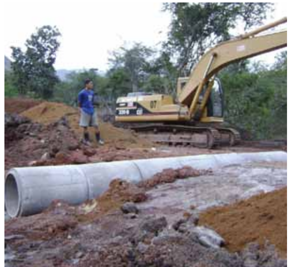
Supporting road construction (Laos)
