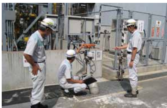
Inspection of dike drainage pump (Oji Paper Co., Ltd. Tomioka Mill)
