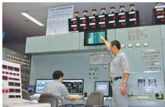
Operators checking warning lights and compliance numbers (Oji Paper Co., Ltd. Tomakomai Mill)
