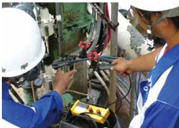
Energy Conservation Patrol checking for waste from air leaks at the Oji Paper Kasugai Mill
