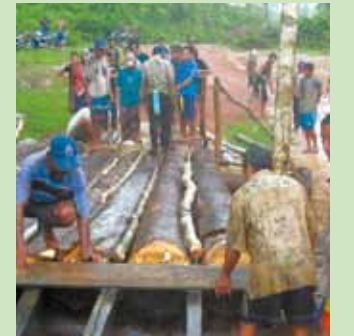
Bridge construction in Nakha Village, Laos
