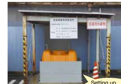
Setting up safety fences around containers for disposal forms part of our leak preparedness measures
