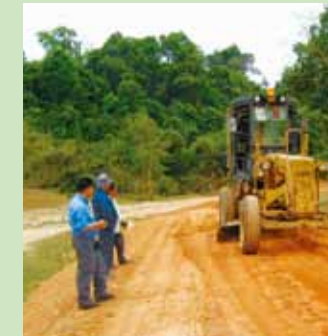
Road construction in Thong Noy Village, Laos
