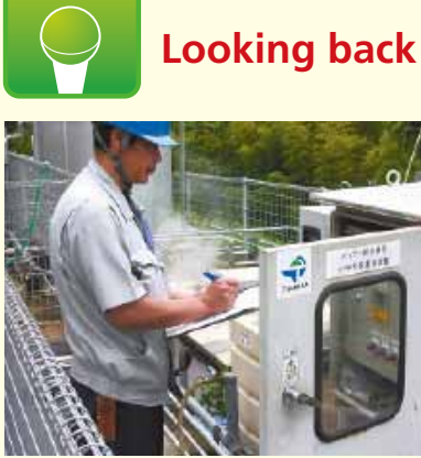
Inspection of wastewater neutralizing equipment
