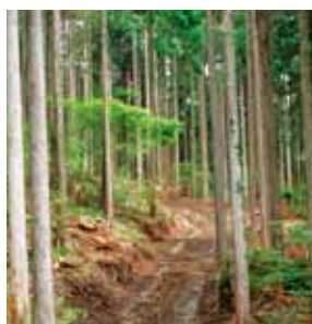
Newly built forest road
