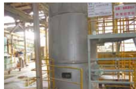
Specialized equipment for difficult-to-process recovered paper (kneading pulper)
