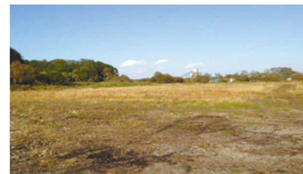
The construction site in Shiranuka Town
