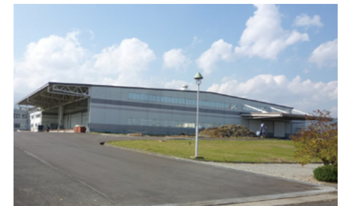
Fukushima Plant (scheduled to begin operations in April 2013)
