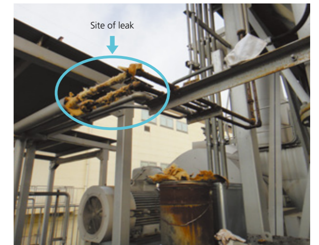
Measures were rolled out after a heavy oil leak was detected from a pipe
