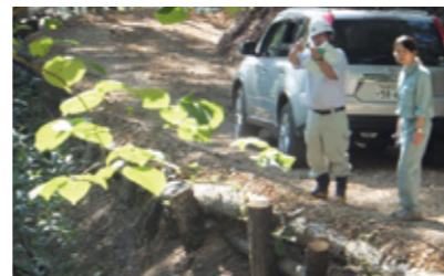
We use logs to shore up work roads
