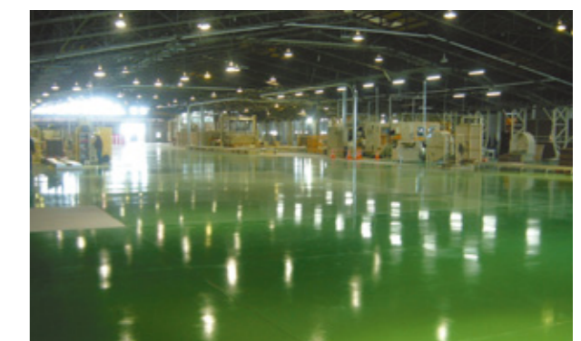
The Sendai Mill after operations were restarted
