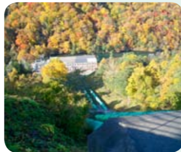
Hydropower generation (see P. 45)
