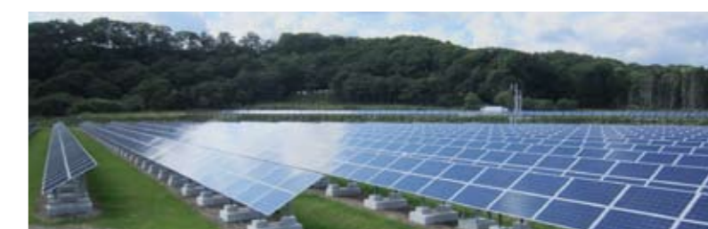
New photovoltaic power generation facility (Oji Green Resources / Shiranuka, Hokkaido)
