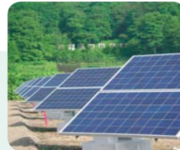
Photovoltaic power generation (see P. 45)
