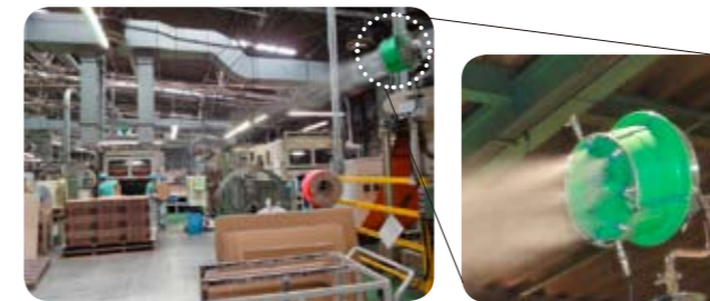
Installation of a mist shower system
