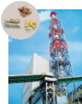
Photo 1 (Inset) RPF made from paper and plastic. (photo) RPF boiler at the Tomakomai Mill of Oji Paper Co., Ltd.
